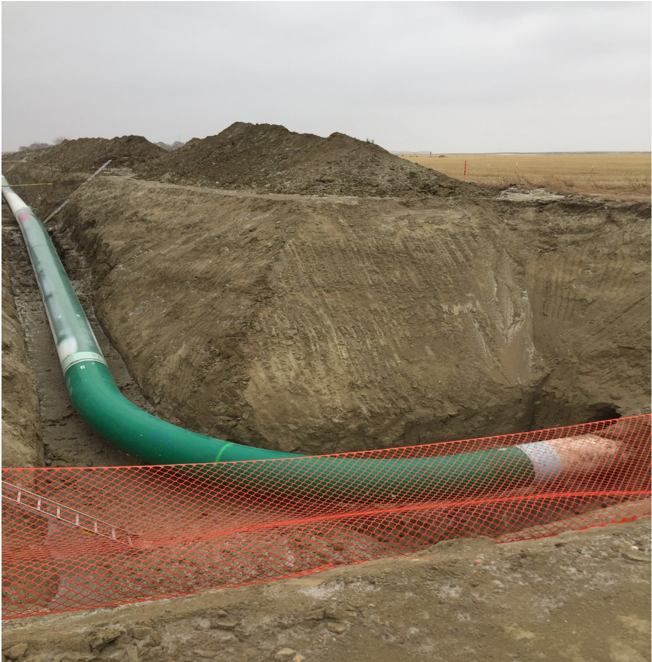
PIPE IN TRENCH WITH A HOT BEND IN IT
