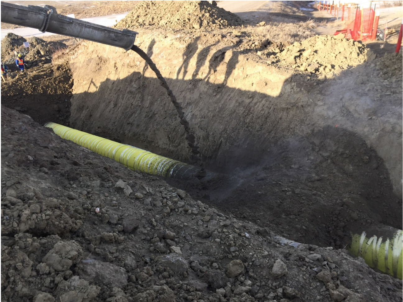
CEMENT TRUCK POURING FILLCRETE ON PIPE ACROSS ROADWAY.
