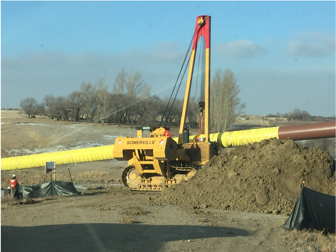
SIDE BOOMS LOWERING PIPE ACROSS ROADWAY.
