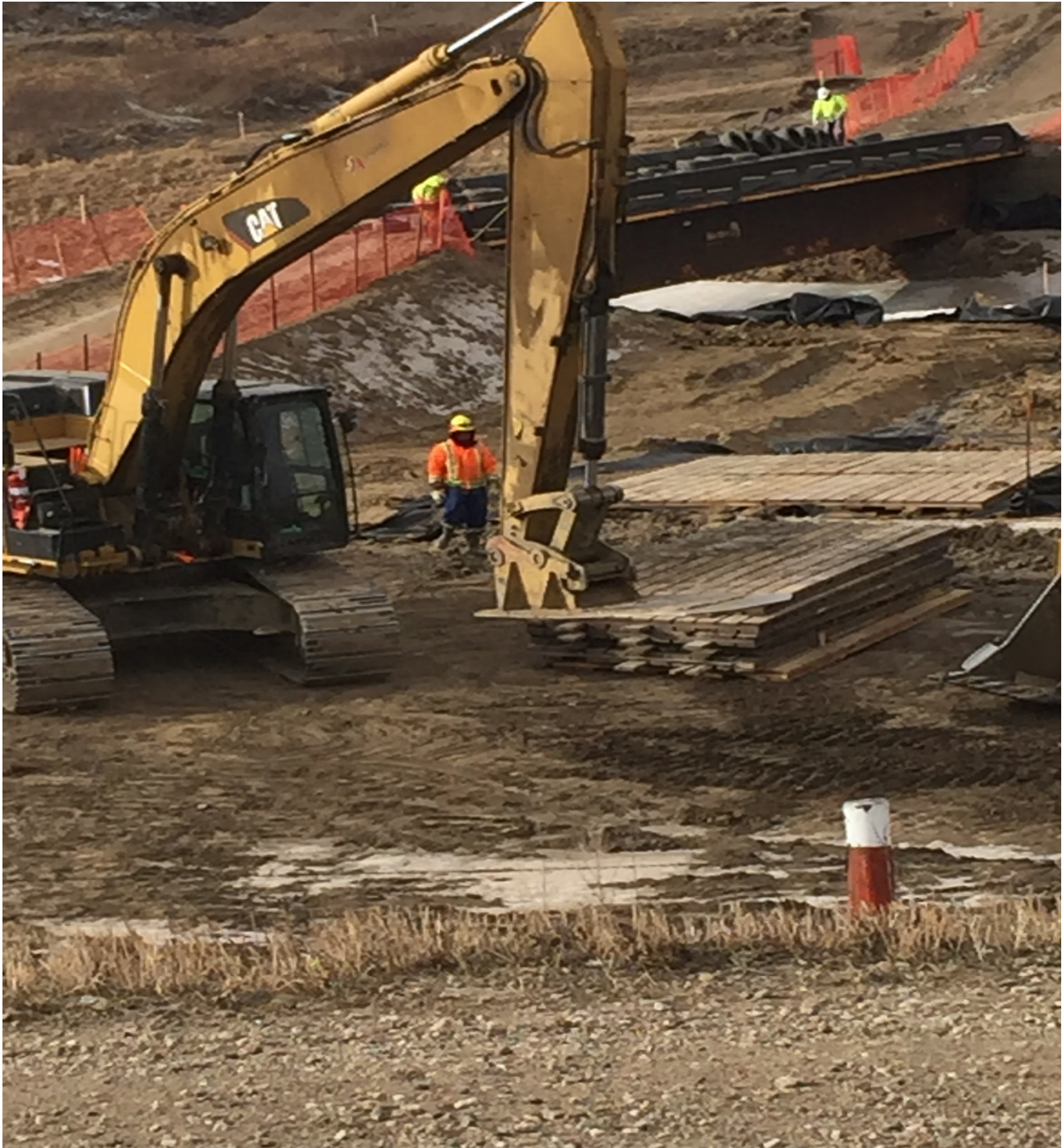
EXCAVATOR LAYING DOWN MATTING BY BRIDGE FOR WALKWAY
