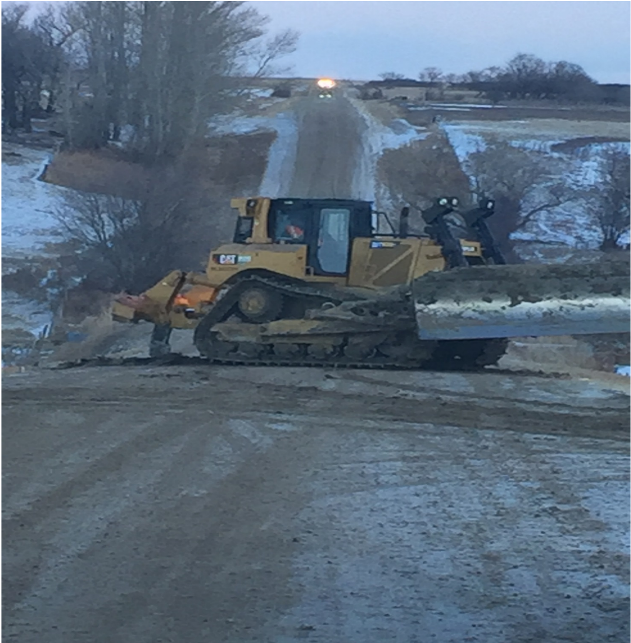
DOZERS RIPPING UP ROAD TO MAKE OPEN CUT.
