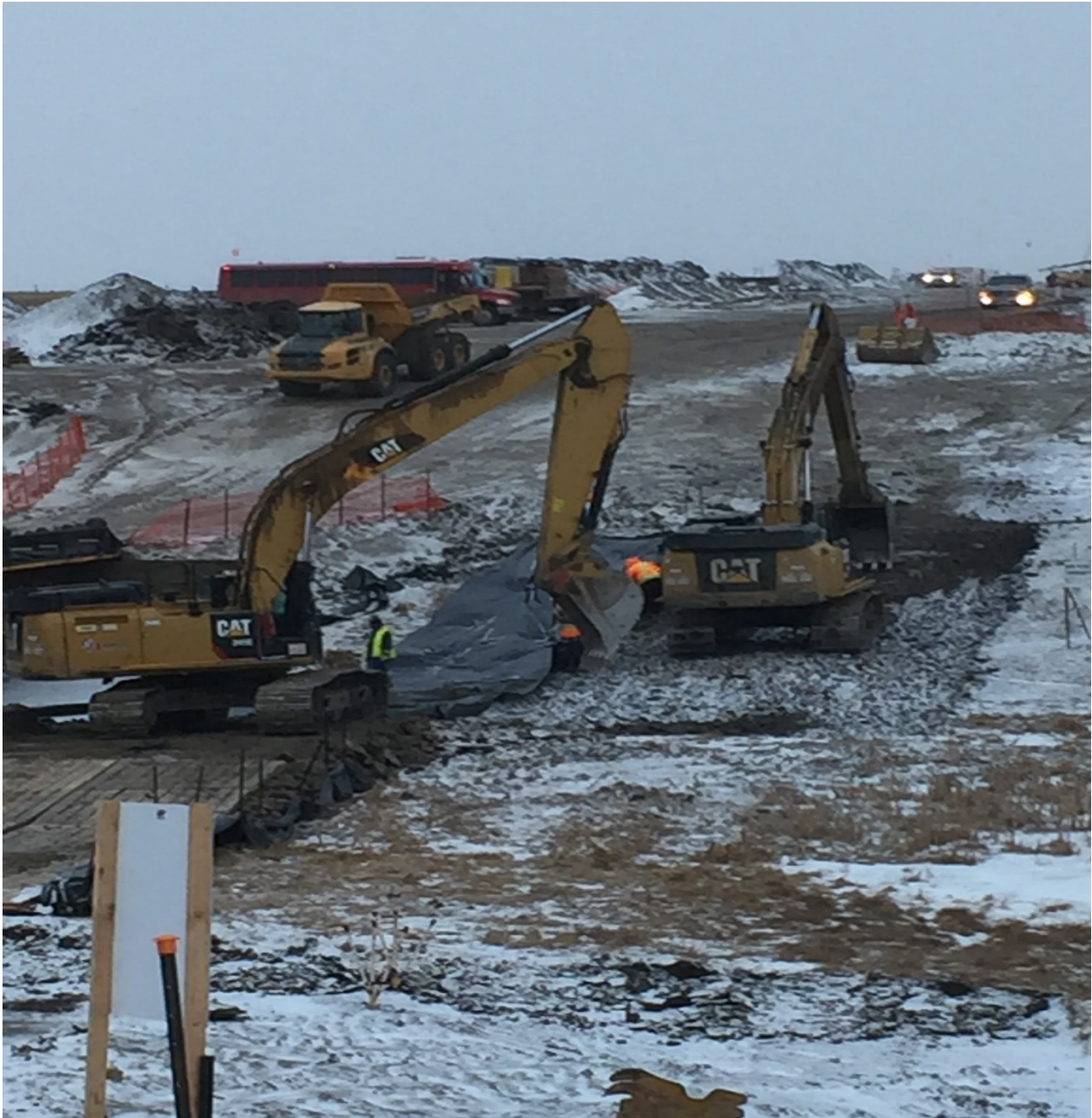
LAYING DOWN GEO TO PRESERVE GROUND WHEN FINISHED
