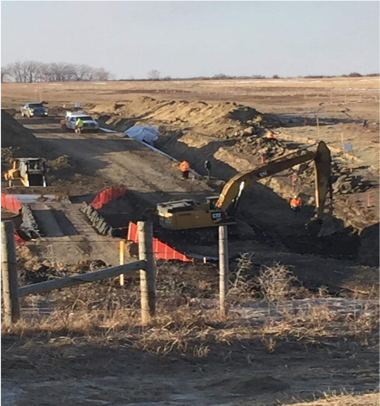
EXCAVATORS DIGGING TRENCH AT HIGH HILL CREEK.
