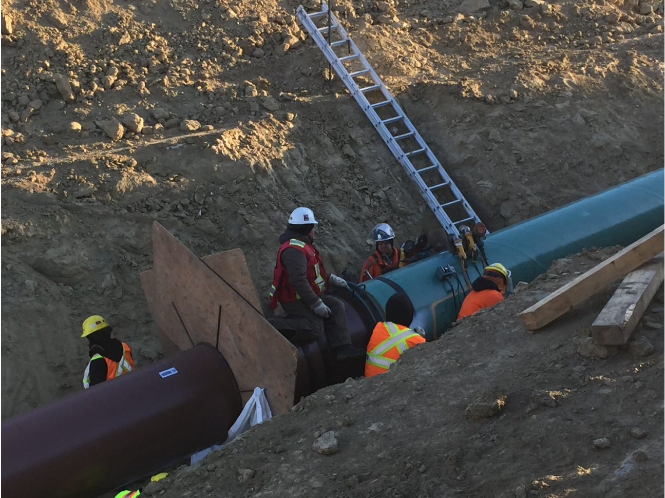
WELDING CREWS COMPLETING TIE-INS.
