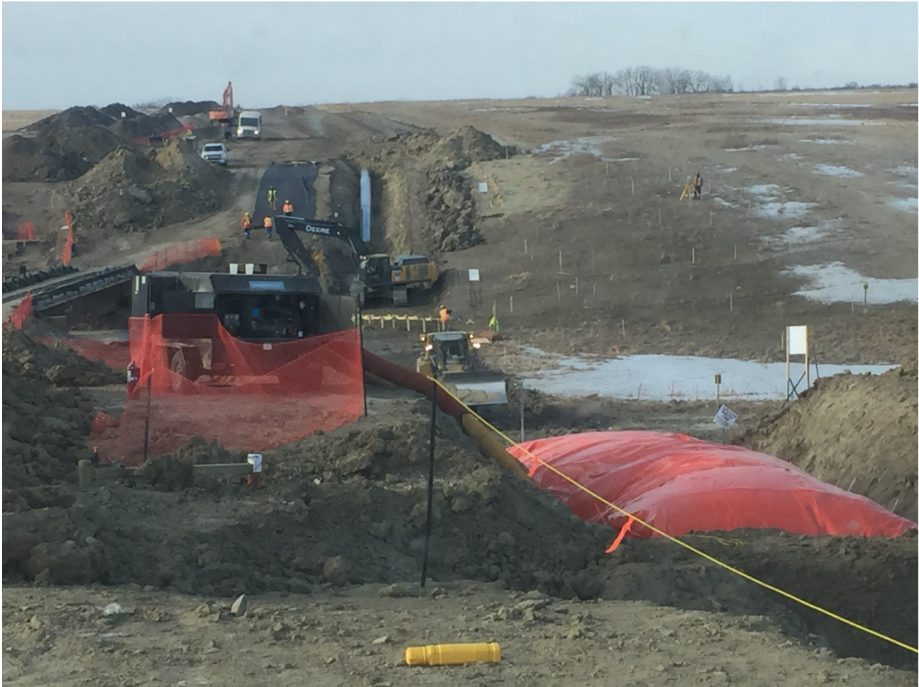
HIGH HILL CREEK WITH OPEN CUT THROUGH ROAD (GENERATOR AND TARP ARE HELPING FILLCRETE SET)
